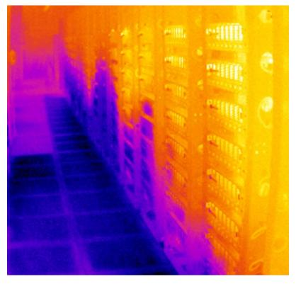
Figure 4) Verifying proper hot aisle/cold aisle operation.
