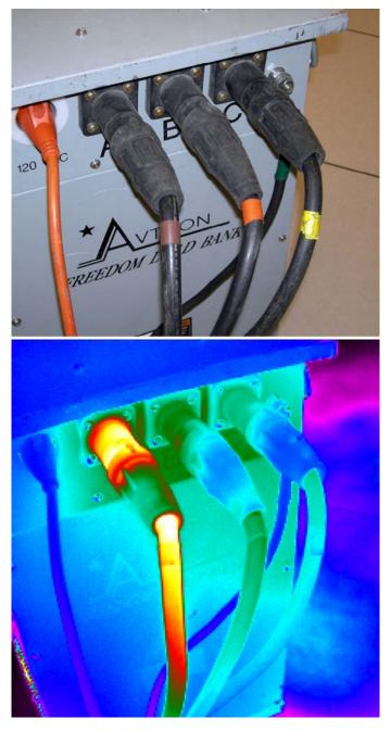
Figure 1) Resistive load bank is shown with a bad cable connection.
