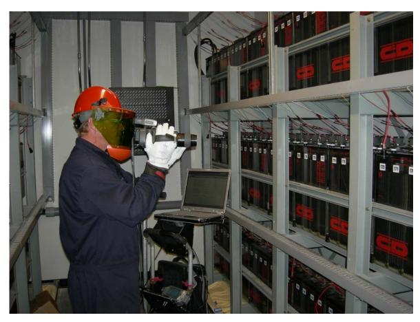
Figure 5) Thermographer inspecting a battery bank during full battery discharge testing.
