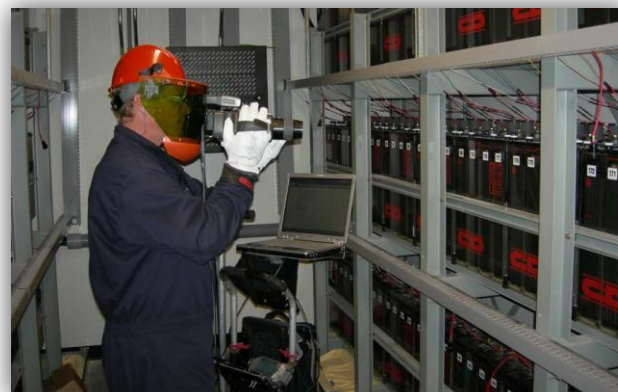
Figures 8a & 8b) Safety around electrical equipment is the #1 consideration during infrared surveying. Some of the options: 8a shows an IRISS infrared window installed in electrical cabinet 5 . The thermographer safely holds an infrared camera up against a viewing port or window to see inside the switchgear. These windows can be custom fit to any data center equipment. 8b) Thermographer wearing proper personal protective equipment (PPE) inspecting a battery bank during a full battery discharge test.
